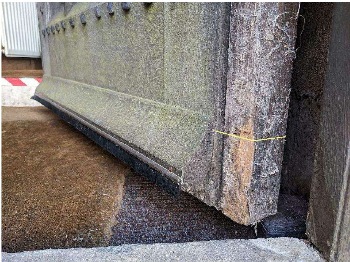
Figure 4 : Base of the oak door, to be trimmed by 100mm and weather bar re-attached
