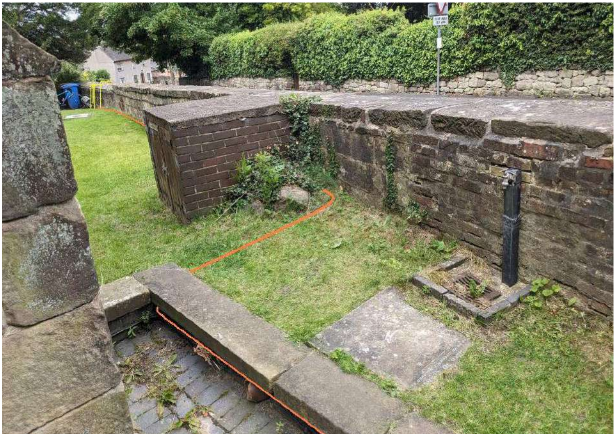
Figure 4 : Cable passes through the gas meter cubicle and into the perimeter gutter
