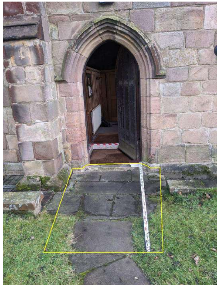
Figure 2 : North door, and extent of proposed ramped paving
