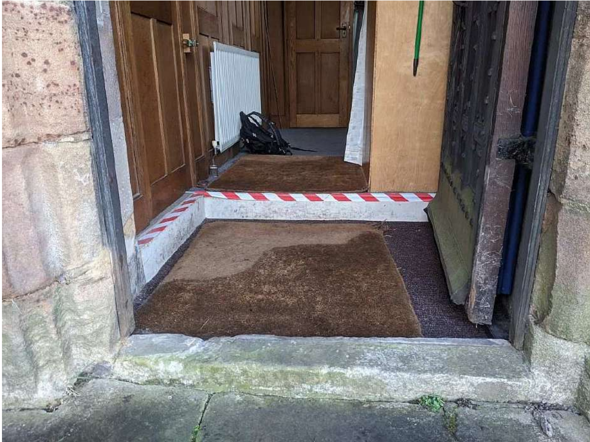
Figure 4 : Base of the oak door, to be trimmed by 100mm and weather bar re-attached
